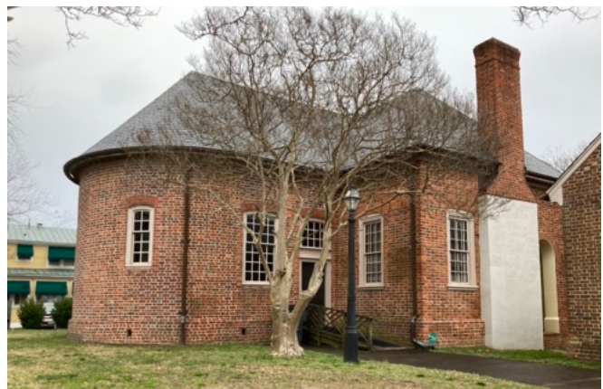
Side and back of 1750 Courthouse
